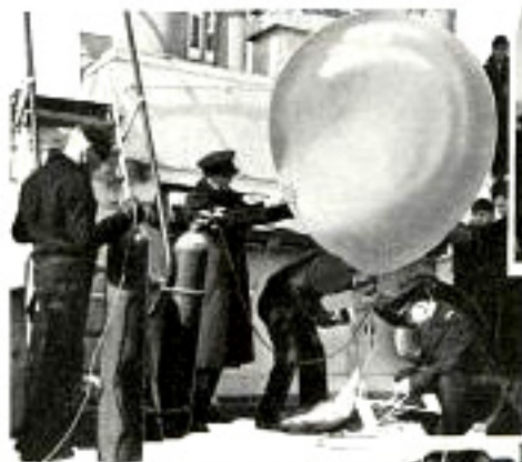
Top, left, Lieutenant Commander Edward M. Smith, commanding the cutter "Chelan," and Lieutenant Ned Strow preparing radio meteorograph for trip aloft; right, sighting departing balloon with theodolite, to compute wind velocity and direction
