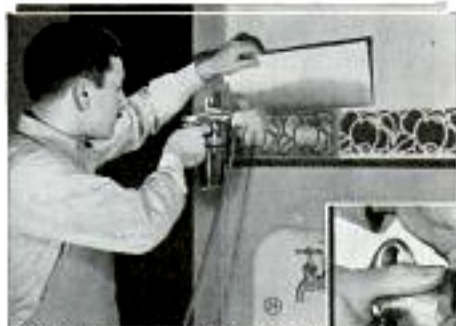
STENCILING IS DONE WITH ROUND SPRAY
