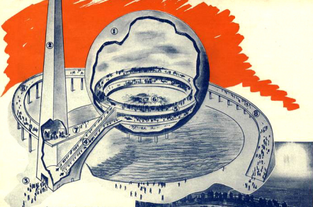
Cutaway drawing shows the Theme Center of the New York World's Fair 1939. This unique twin structure will house the focal exhibit of the Exposition. The drawing shows: 1—Perisphere, a 200-ft. sphere; 2—Tyrlos, a 700-ft. triangular obelisk; 3—Entrance to exhibit; 4—Escalators carrying visitors to 65-ft. level; 5—Revolving platform from which to view the interior; 6—Model of the City of Tomorrow; 7—Exit Bridge leading to descending ramp; 8—Helixline or Exit Ramp enclosing the structures.
