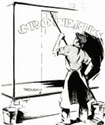
Gutter at bottom of show window drains dirty water into a bucket and keeps it off sidewalk
