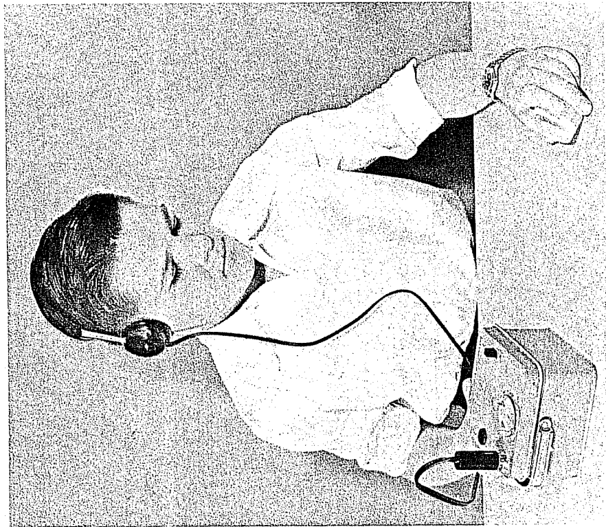
Figure 1-9. EXPERIMENTING WITH THE GILBERT GEIGER COUNTER.
