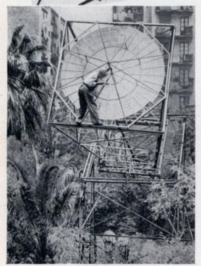
A TRAP FOR OLD SOL. Here a workman is polishing up the prisms of the solar furnace shown above. The tower turns to face the sun
